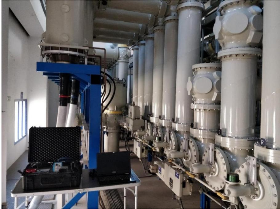
Figure 4. Installation of PD monitoring systems inside a GIS substation.
